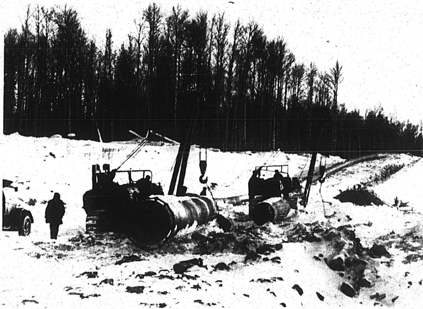
SOVIET GAS LINE — A 1,320-mile gas trunk line is being laid from the Tyumen Region in Western Siberia to the Central area of the country. — NOVOSTI PRESS AGENCY Photo
