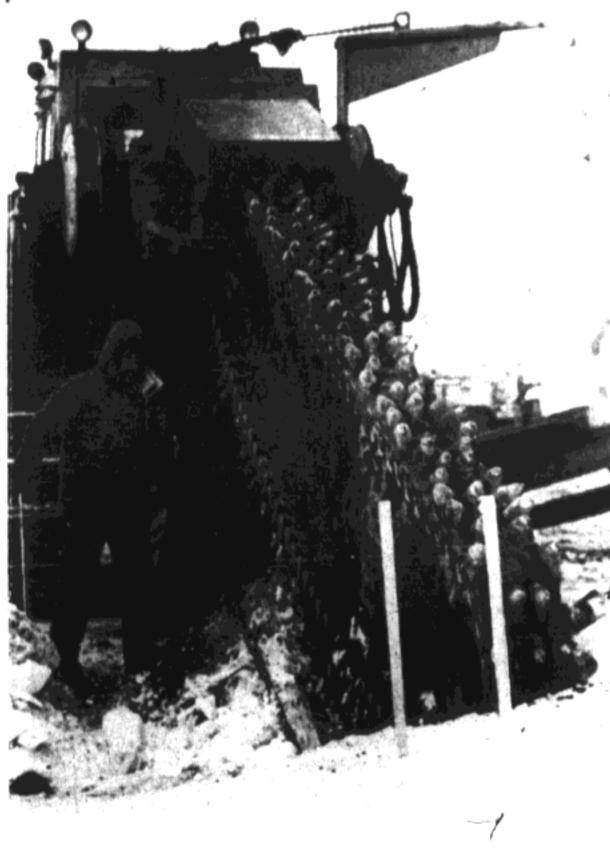
'Wherever it goes, huge square ditches ten feet deep and ten feet wide are required to bury the utilidor. You don't dig such a ditch. You cut it. To do that the North Slope Borough has enlisted a large rock saw that looks like a chain saw for King Kong stuck on a bulldozer."
