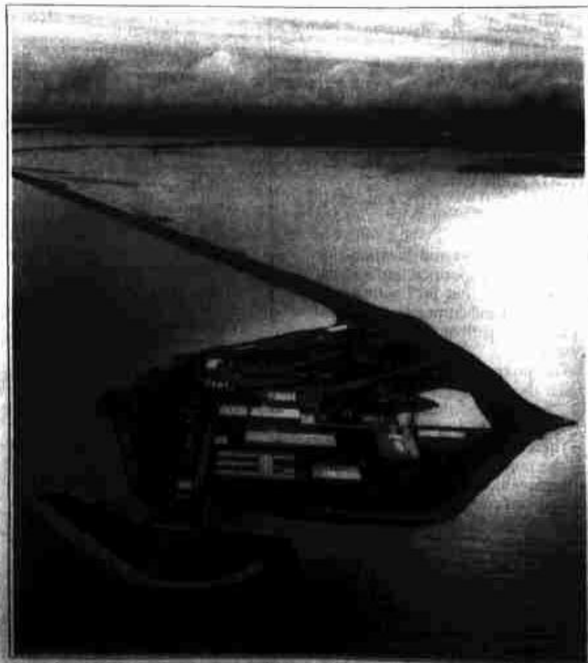
The 45-acre Main Production Island is shown in the foreground. It is connected to a satellite drilling island and the shore with a 5-mile causeway.
