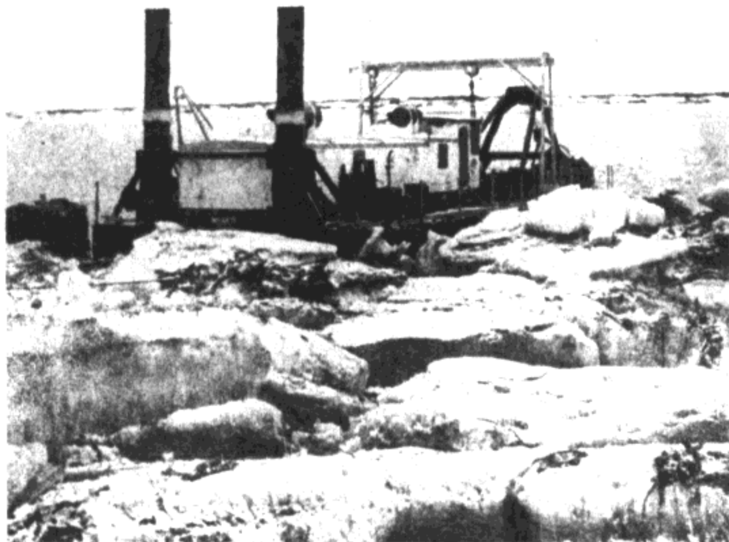
The dredge Nuvakti waits for break-up on the Colville River near Nuiqsut. This dredge brought up the gravel that made the award-winning new airport for the village east of Barrow.
