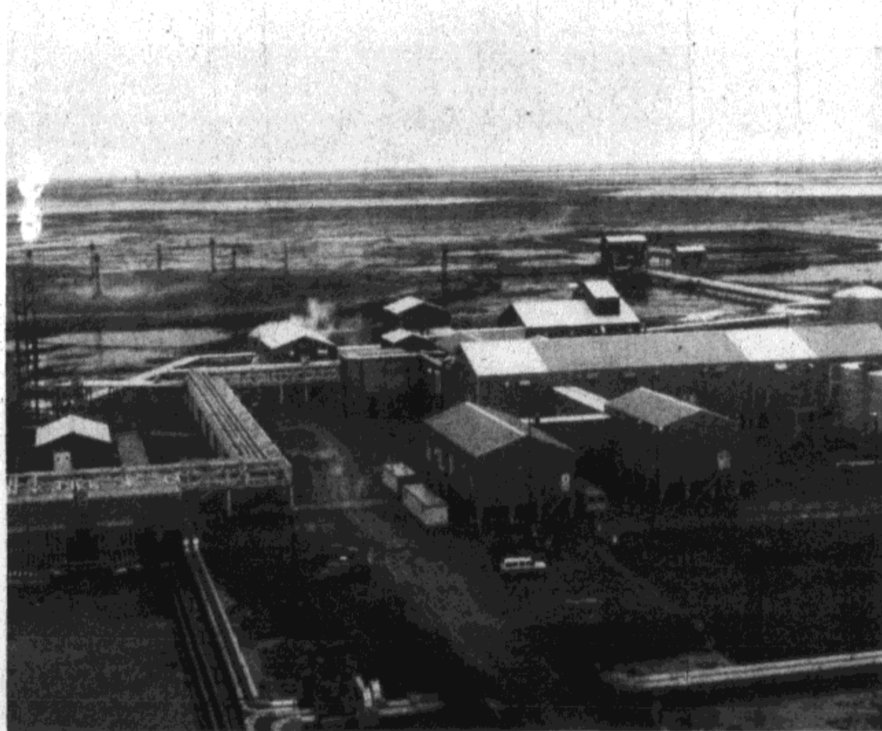
Atlantic Richfield's central compression plant and field fuel gas unit supplies the field with gas for fuel.
