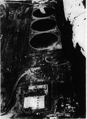
CONSTRUCTION IS UNDER WAY on three ballast water storage tanks at the Valdez terminal for the 800-mile-long trans Alaska pipeling. The tanks, which will have a capacity of 430,000 barrels, will receive ballast water from tankers for treatment to remove pollutants. Foundations are being poured for a ballast treatment building bottom.
