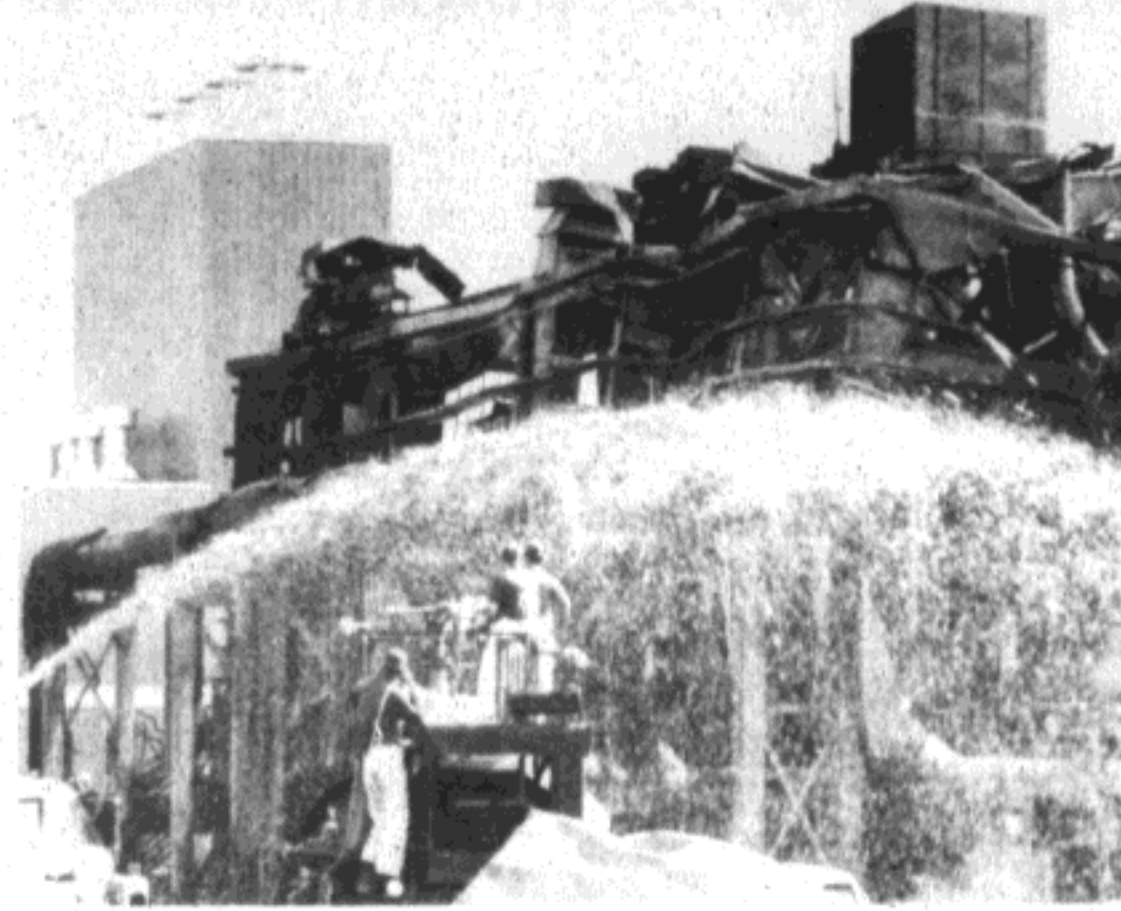
DEVASTATION AT PUMP STATION 8 — Flame retardant is sprayed on the still hot, smouldering debris of the totally destroyed main pump building.
