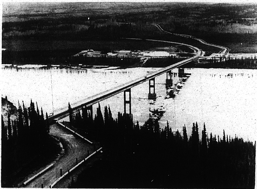
THE TRANS-ALASKA PIPELINE is to cross the Yukon River on a special pipeway built aside the 2,300-foot-long Yukon River Bridge completed in the fall of 1975. Pipe laying on the bridge is scheduled for later this summer.
