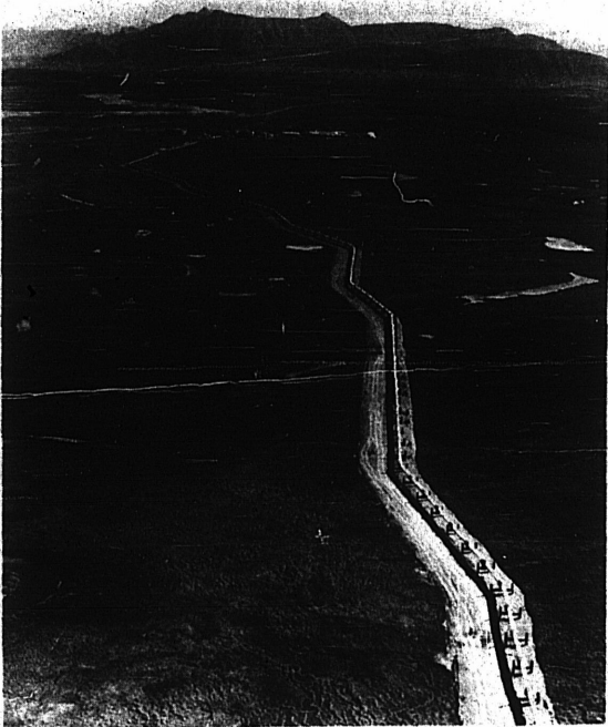
The gravel and insulation workpad underlying the trans Alaska pipeline on Alaska's North Slope near Pun Station 3 prevents degradation of subsurface permafrost.
