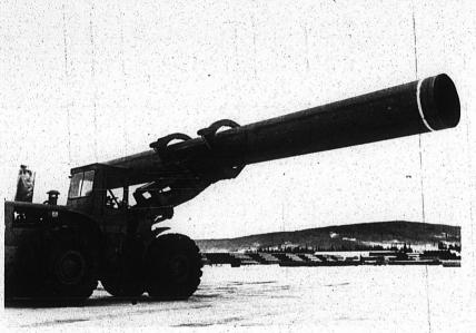
IT'S NOT REALLY Alaska's version of the "Big Bertha" cannon . . . it's a 60-foot-long section of pipe at a pipe storage yard in Fairbanks. The 48-inch-diameter pipe for the trans-Alaska pipelline is being readled for shipment to points along the 798-mille-long pipelline route. Full-scale pipelline construction is expected to be under way in the early spring of 1975.
