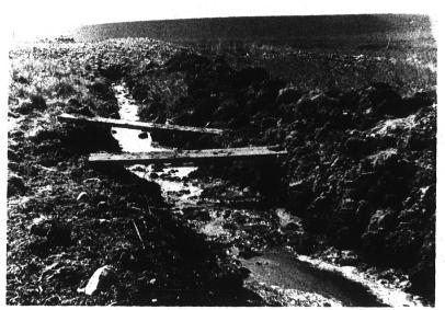
LIMITED SUCCESS IN CLEAN-UP ATTEMPT— A fuel oil leak inside a utility building at the Happy Valley pipeline construction camp and a new leak this June continue to cause problems. "The cut-off trench below the waste area had only limited success in stopping the sub-surface
