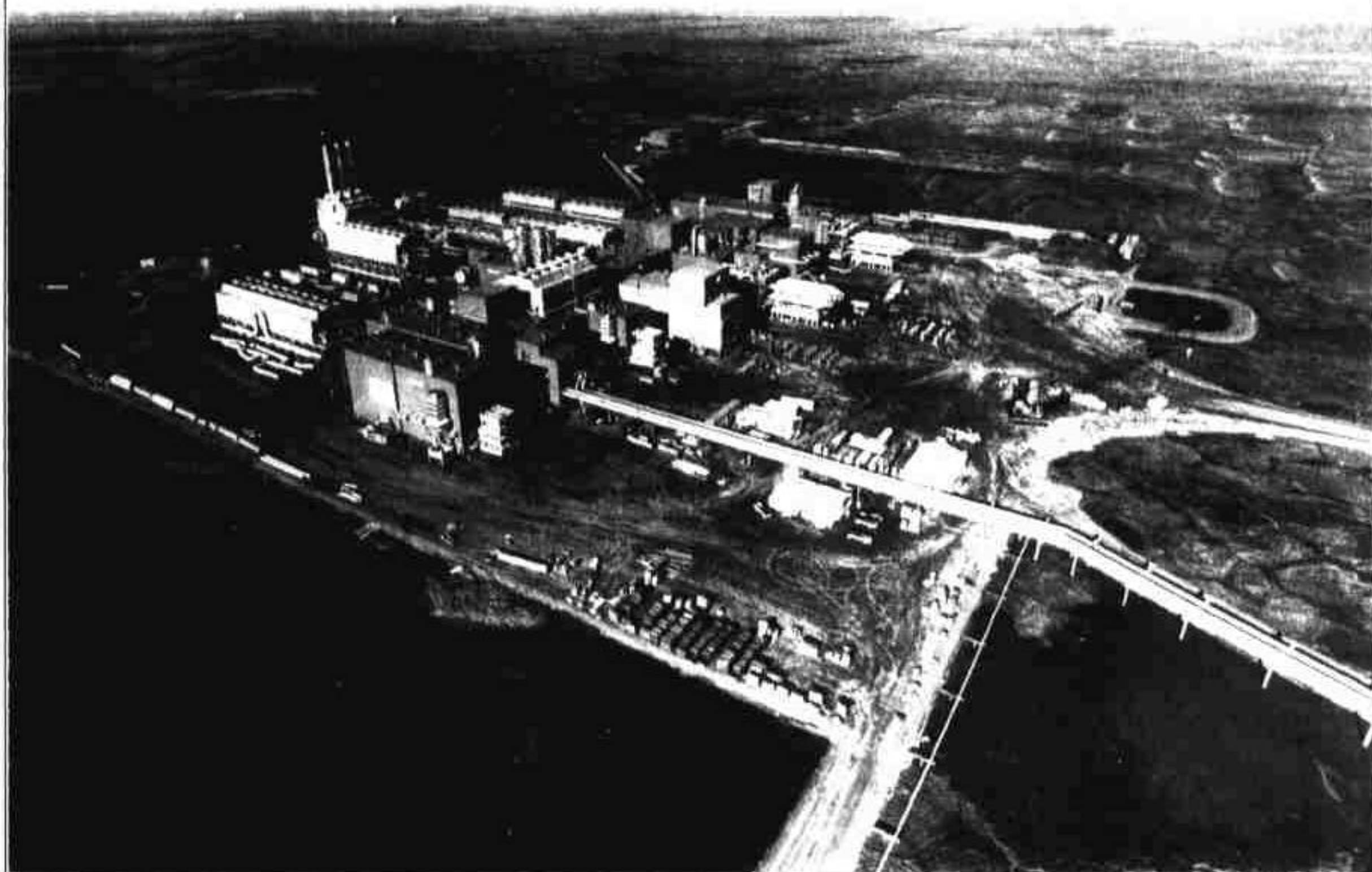
Prudhoe Bay's new Central Gas Facility, now in operation, soon will be producing more than 40,000 barrels of natural gas liquids. The plant removes natural gas liquids from the natural gas stream and blends them with the crude oil stream in the trans Alaska pipeline.
