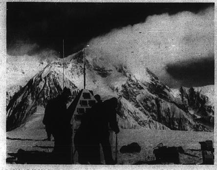
RADIO AT 13,700 FEET—The Bureau of Land Management radio repeater station is being put up at one of Mt. McKinley's northwest peaks at 13,700 foot level. Two technicians, Roger Wirch, left, and John Senn, are finishing up the anchor-
