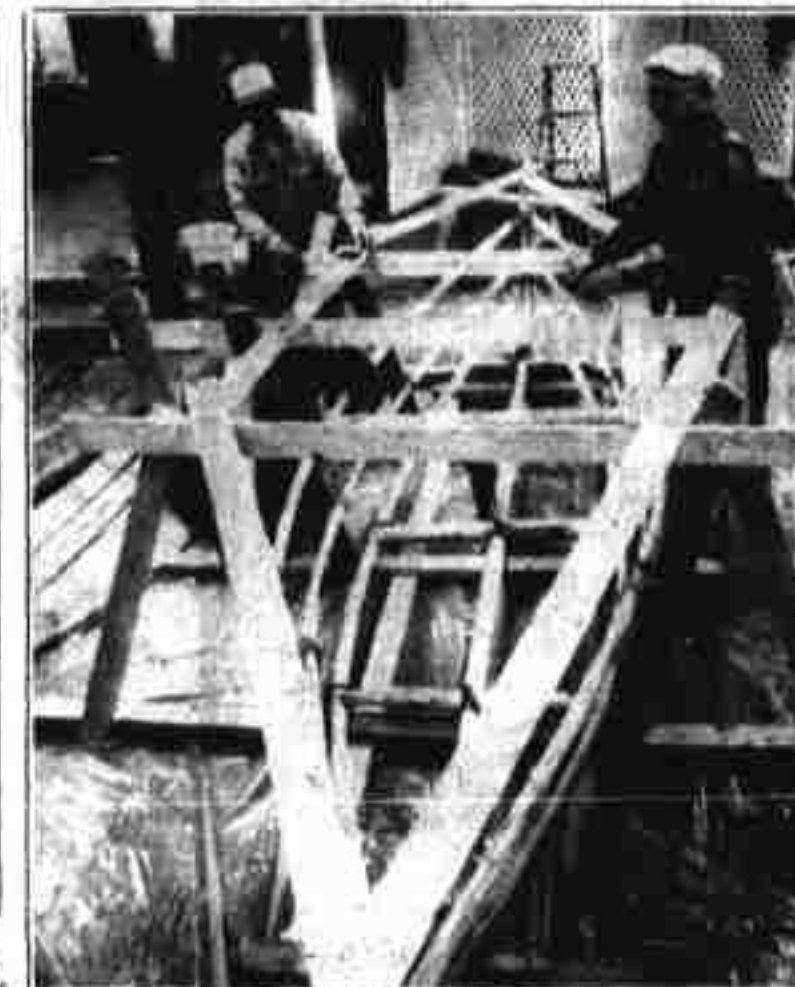
The canoe frame is 16 and a half feet long, 4 feet wide at the top, 3 feet wide at the bottom and 20 inches deep.
