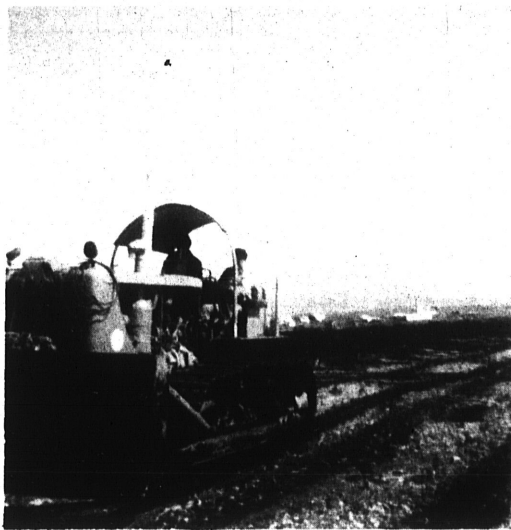
BIG CAT MAKES TRACKS ON NEW AIRFIELD — Driver Lynn Peterson instructs Nick Peterson in Operation of the D-8 tractor being used to clear the new runway at Akhiok. The machine was acquired through the RurAL CAP VEMP program.
