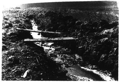
LIMITED SUCCESS IN CLEAN-UP ATTEMPT-A fuel oil leak inside a utility building at the Happy Valley pipeline construction camp and a new leak this June continue to cause problems. "The cut-off trench below the waste area had only limited success in stopping the sub-surface
